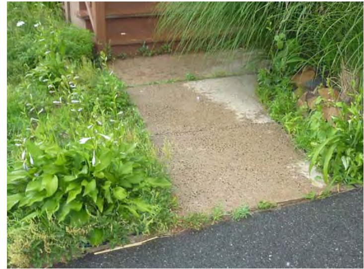
Trip hazard at asphalt/concrete paving joint and at irregular height stair risers are shown to be eliminated in Year 1.
