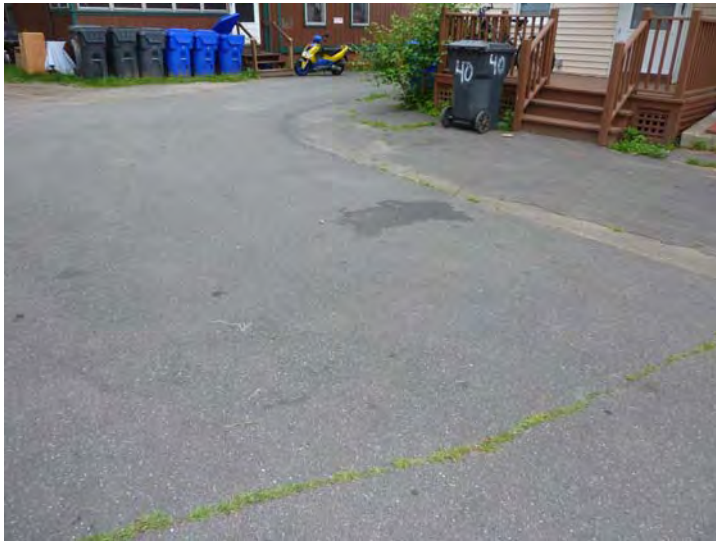
Typical cracking of asphalt paving in project drive. Crack seal is shown in Year 1.
