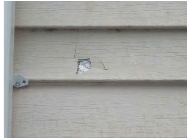
Typical localized vinyl siding damage.
