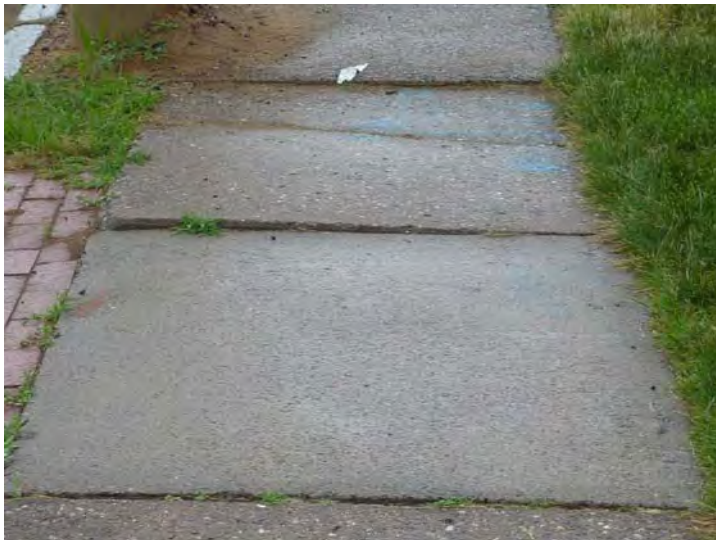
Typical trip hazards at concrete walks are shown to be eliminated in Year 1.
