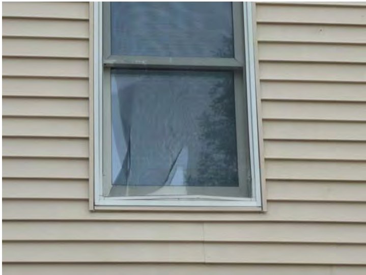
Typical screen damage. Obtaining replacement screens is not possible, resulting in insurance issues.
