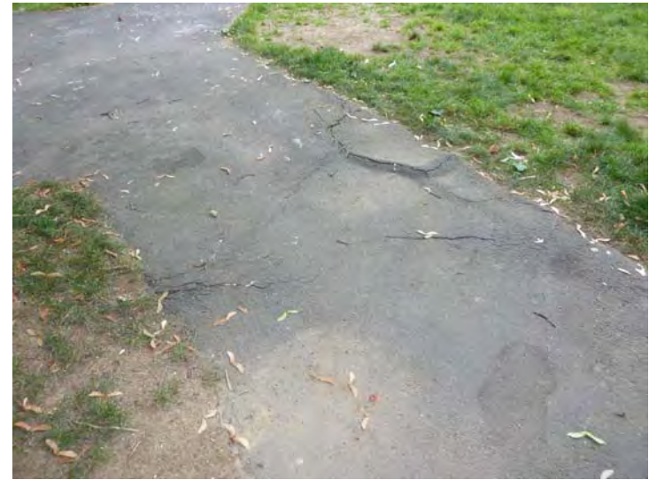
Asphalt walk damage from adjacent tree roots is shown to be replaced in Year 1.
