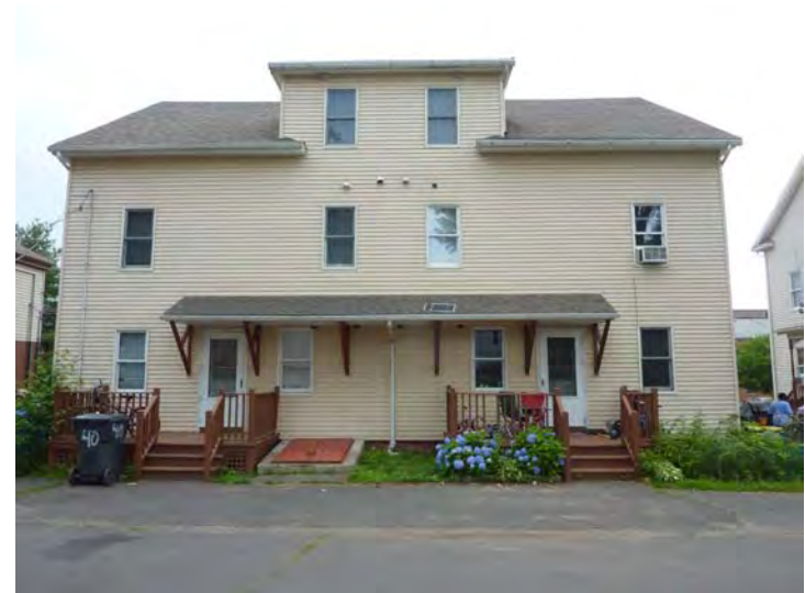
Typical wood decks and stairs at rear are shown to be repaired and painted regularly. Roofing is shown to be replaced early in the plan based on EUL and condition.
