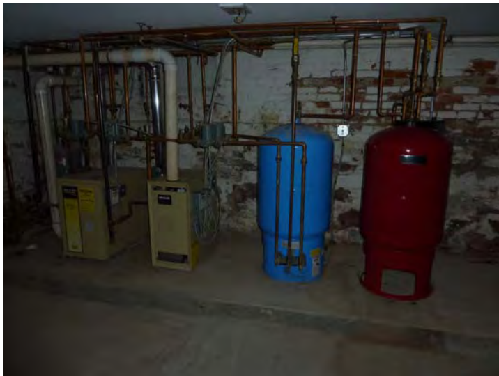
Typical gas-fired hot water boilers, domestic hot water heater and storage tank in each building basement.
